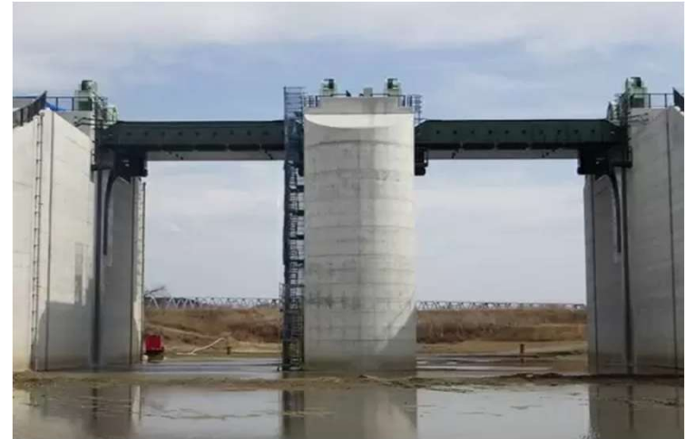
Figure A-1-11: Nagashima water gate (horizontal roller gate)
