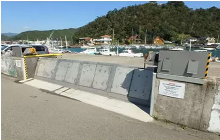
Figure A-1-12: Flap gate-type movable sea wall installed on land
