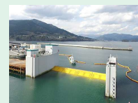
Flap-Gate Type Seawall against flood disaster
