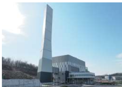
HirakataKyotanabe Regional Flammable Waste Treatment Facility (Kyotanabe City, Kyoto Prefecture)
