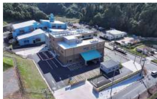
Kanadevia Narita Purification Center (Narita City, Chiba Prefecture)
