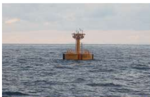
Marine observation equipment for Fisheries environment improvement work in Muroto
