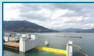
Flap-Gate Type Seawall Against flood disaster
